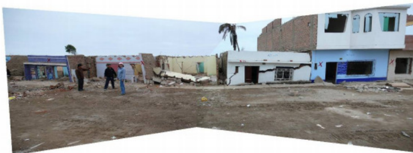
Fig. 3.25. Settlement of 0.7 m of building in front of palm tree.
